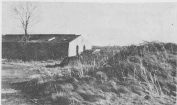
Remains of old hardstand in foreground
