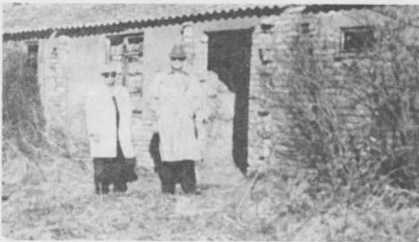
Old crew quonset?
