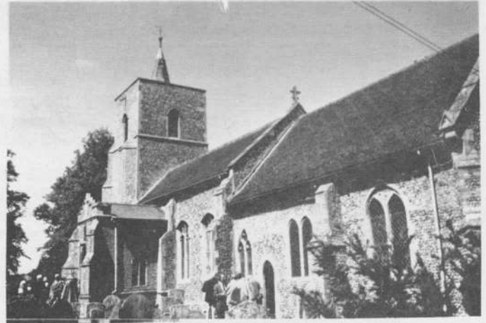
We helped with the roof repair for "our" Church
