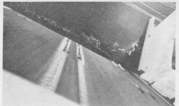
Looking down the spillway at Grand Coulee Dam
