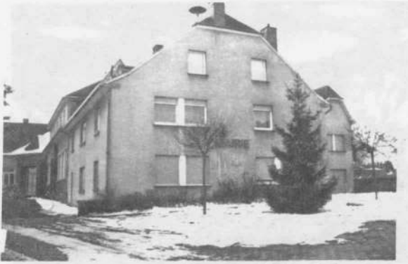
First floor of this school in Perle Luxembourg will house our 385th Museum that Roger Feller is developing.
