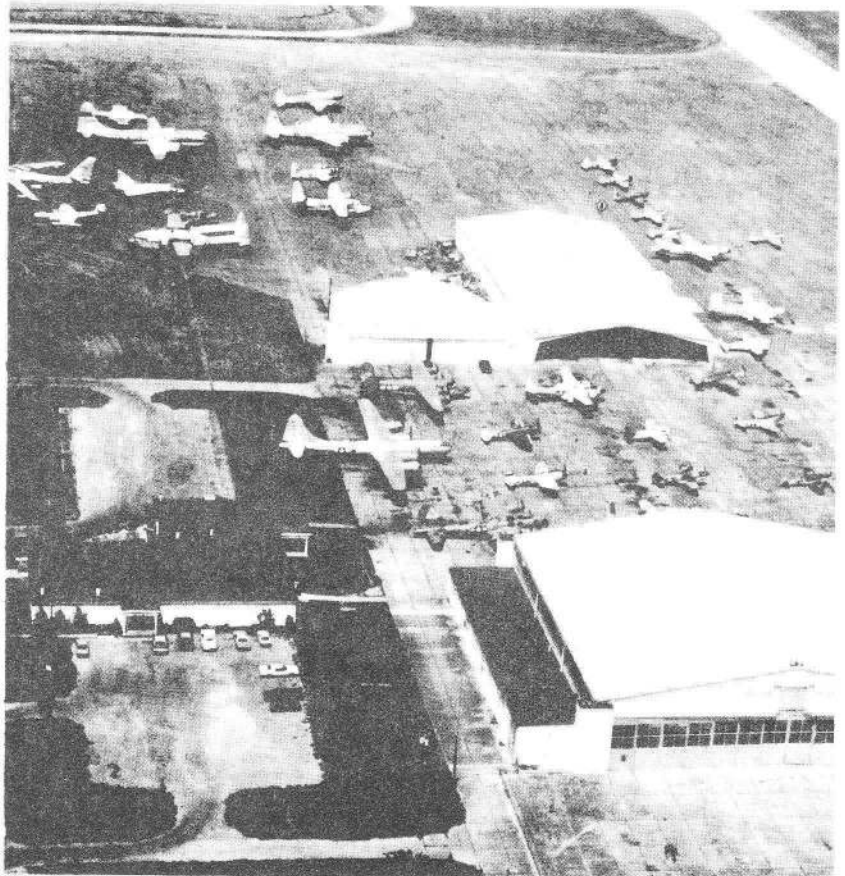
Home of the CAF at Rebel Field — lower right: bomb wing hangar; lower left: indoor museum, CAF offices and officers club; upper right: fighter wing hangar and maintenance hangar; top left: static display area.
