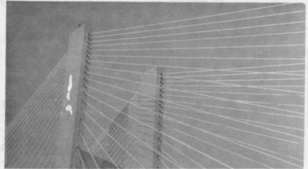
The Suspension Bridge
