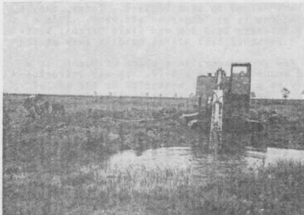
Debris scattered around after digger made first sweep..
