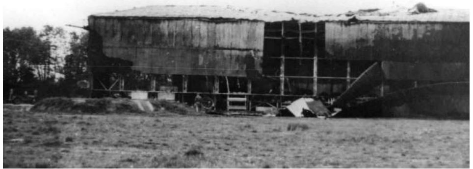
Great Asfield May 23, 1944 - Side Blown Off #1 Hangar
