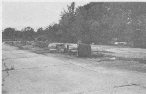
Site of hanger No. 1 at Great Ashfield.
