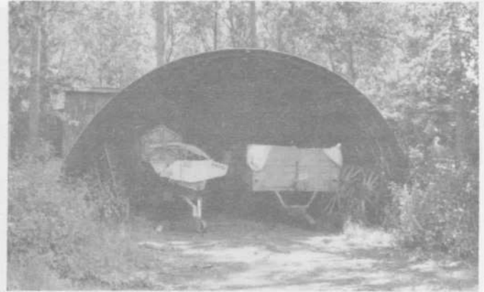
Quanset Hut, now being used to store farm equipment
